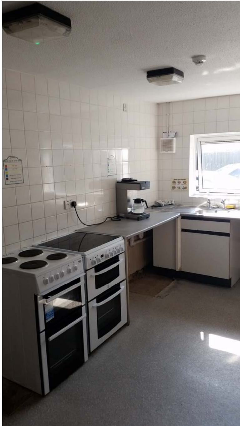
Photo. 7 – General view of GF main kitchen area.
