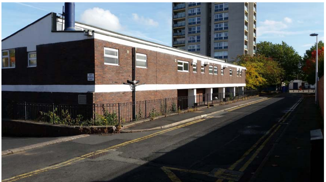
Photo. 2 – General view of Belvedere and front entrance.
