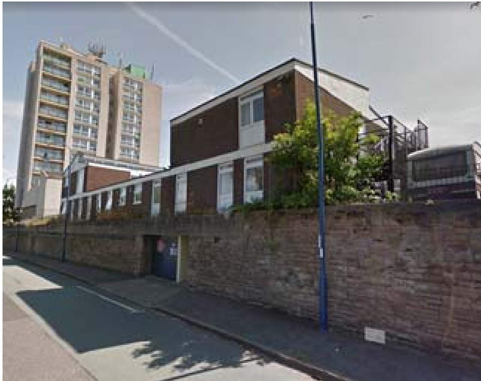
Rear Elevation – Note basement car park entrance.
